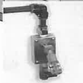
Surface Mount air line is mounted to the wall
